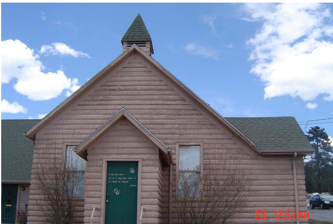
Figure 2: Schoolhouse section, camera facing north, April 23, 2009; OAHP files, photographer: Heather Peterson
