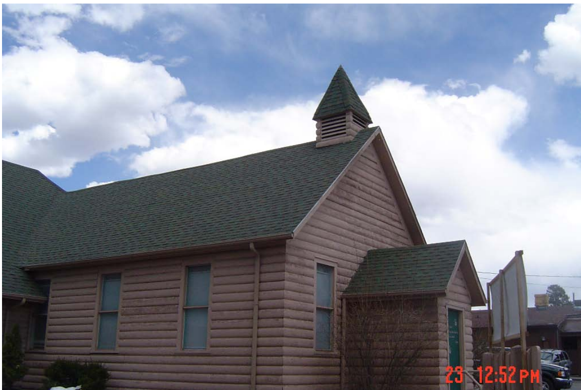
Figure 3: Schoolhouse section, camera facing northeast, April 23, 2009; OAHP files, photographer: Heather Peterson
