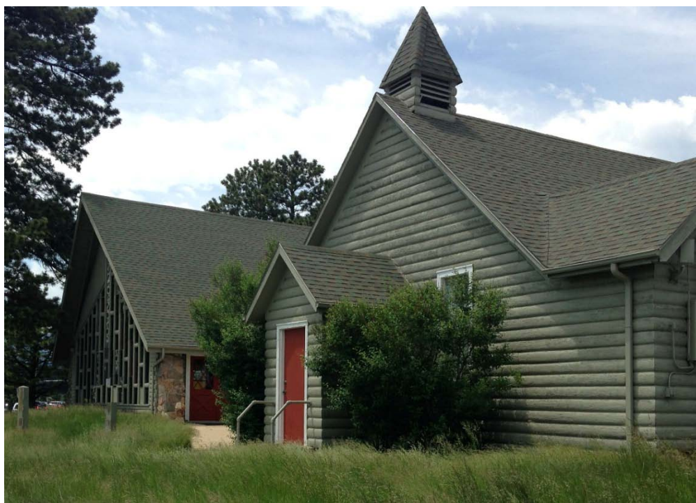
Figure 12: East-facing side, prior to rehabilitation, 2017, camera facing northwest, photographer: Rome Chelsi
