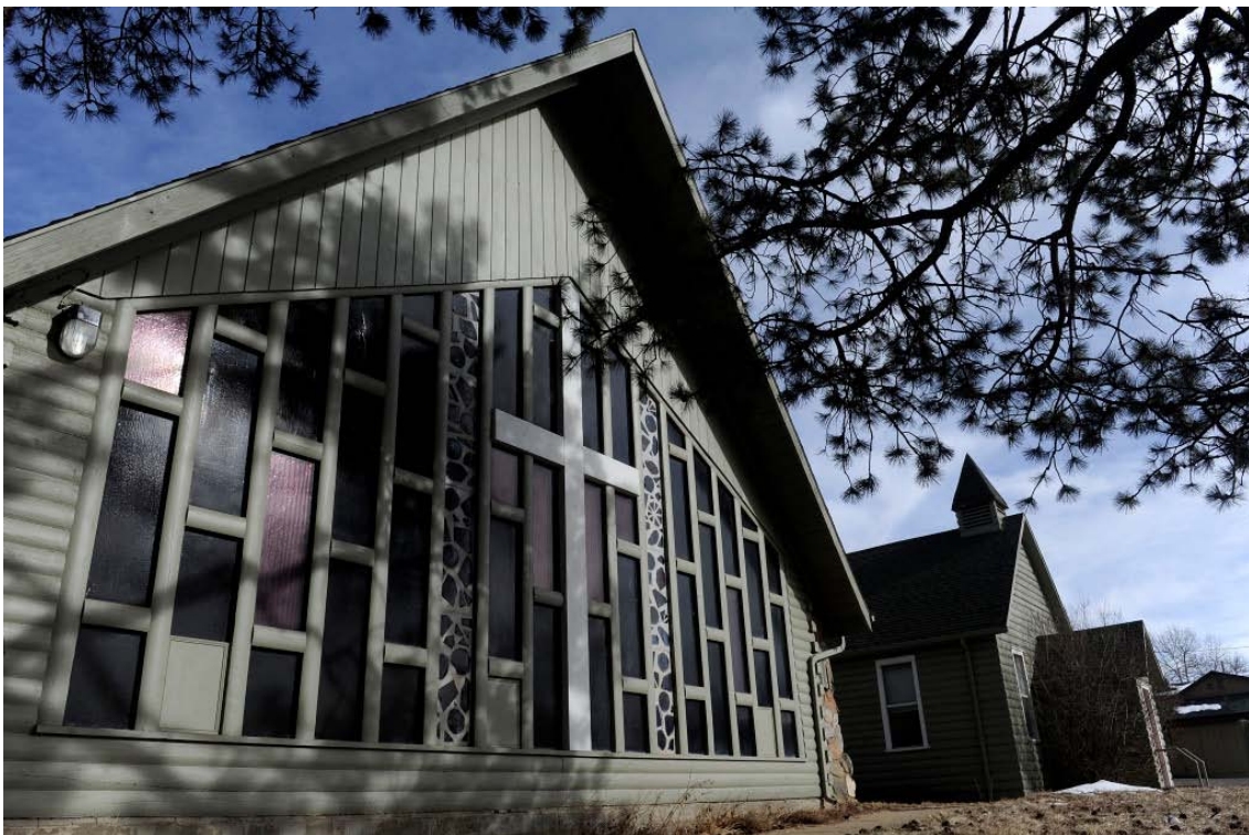
Figure 11: Sanctuary, east-facing side, camera facing northeast, prior to rehabilitation, ca. 2016, unknown photographer
