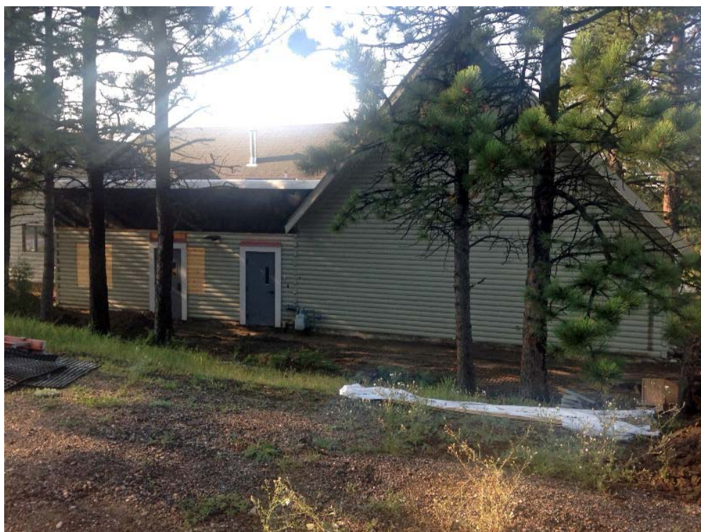
Figure 13: North-facing (rear) side, during rehabilitation, 2017, camera facing south, photographer: Rome Chelsi
