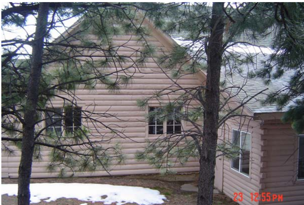
Figure 9: Schoolhouse, north-facing side (rear), camera facing south, April 23, 2009; OAHP files, photographer: Heather Peterson
