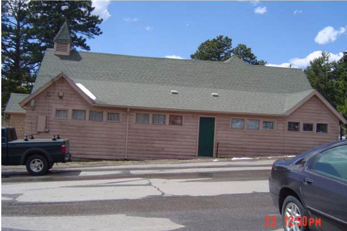
Figure 10: Schoolhouse, east-facing side, camera facing west, April 23, 2009; OAHP files, photographer: Heather Peterson
