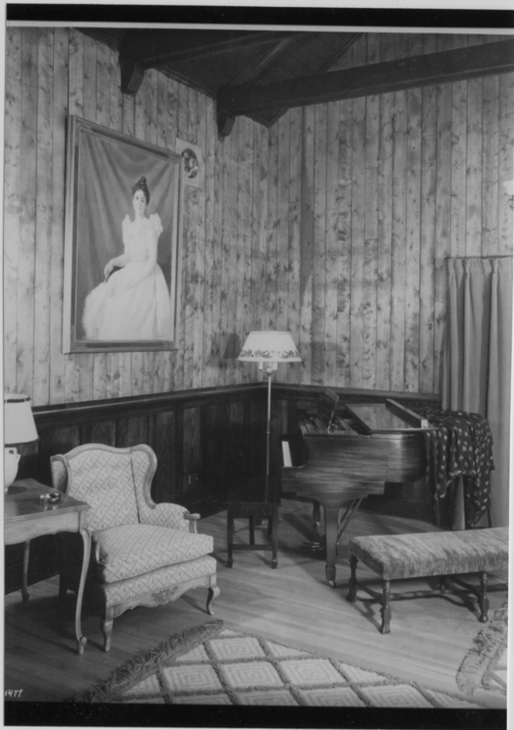
1935 Northwest corner of main room
