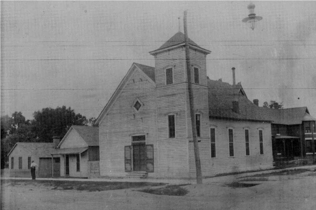
Figure 1: Eighth Street Baptist Church ca. 1905, east and north sides. (Image included in site file held by History Colorado Office of Archaeology and Historic Preservation, original source unidentified; also reprinted in They All Came to Pueblo: A Social History )
