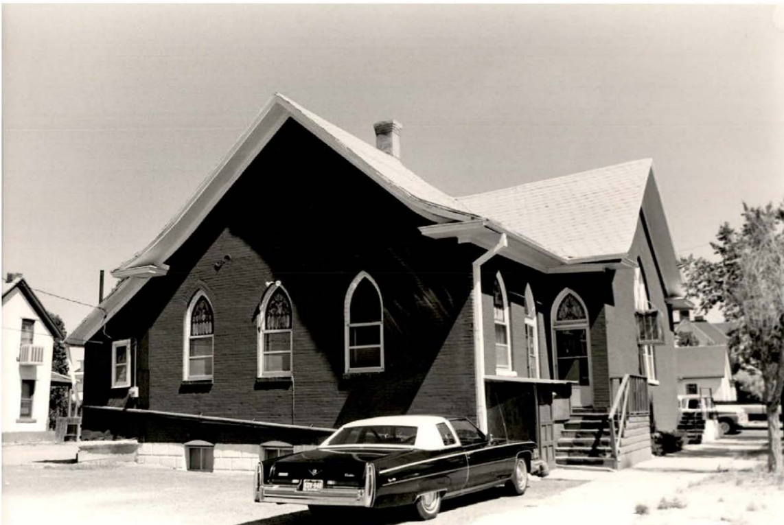
Figure 16: Eighth Street Baptist Church, June 1985, south side. (Jim Munch, Pueblo Department of Planning and Development/ History Colorado Office of Archaeology and Historic Preservation site files, 5PE.1228)
