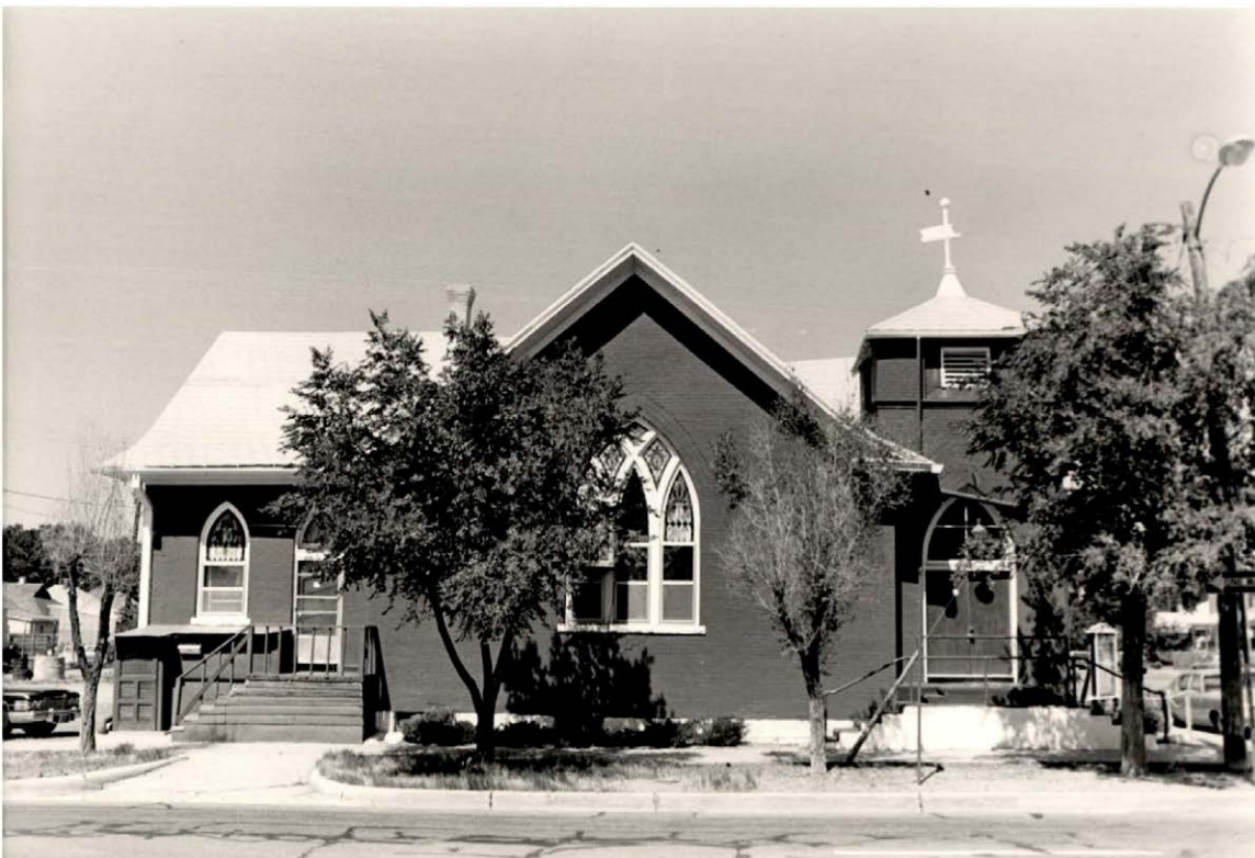
Figure 14: Eighth Street Baptist Church, June 1985, east side. (Jim Munch, Pueblo Department of Planning and Development/ History Colorado Office of Archaeology and Historic Preservation site files, 5PE.1228)
