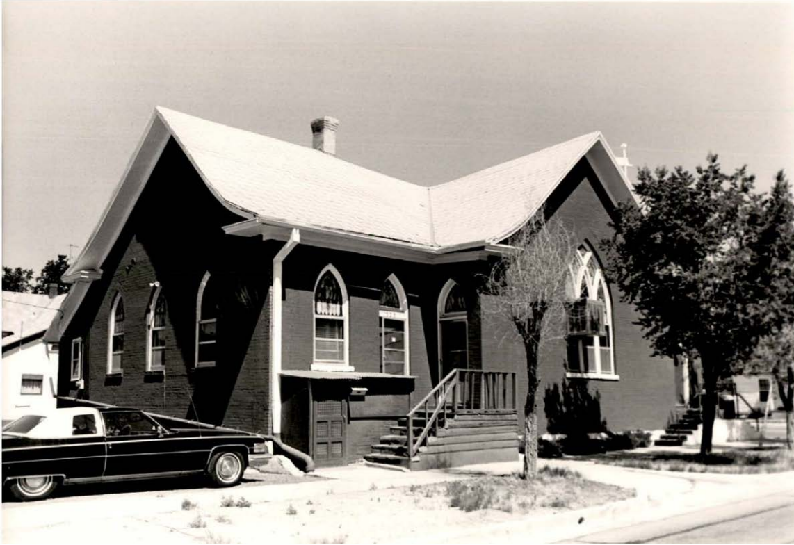
Figure 15: Eighth Street Baptist Church, June 1985, south and east sides. (Jim Munch, Pueblo Department of Planning and Development/ History Colorado Office of Archaeology and Historic Preservation site files, 5PE.1228)
