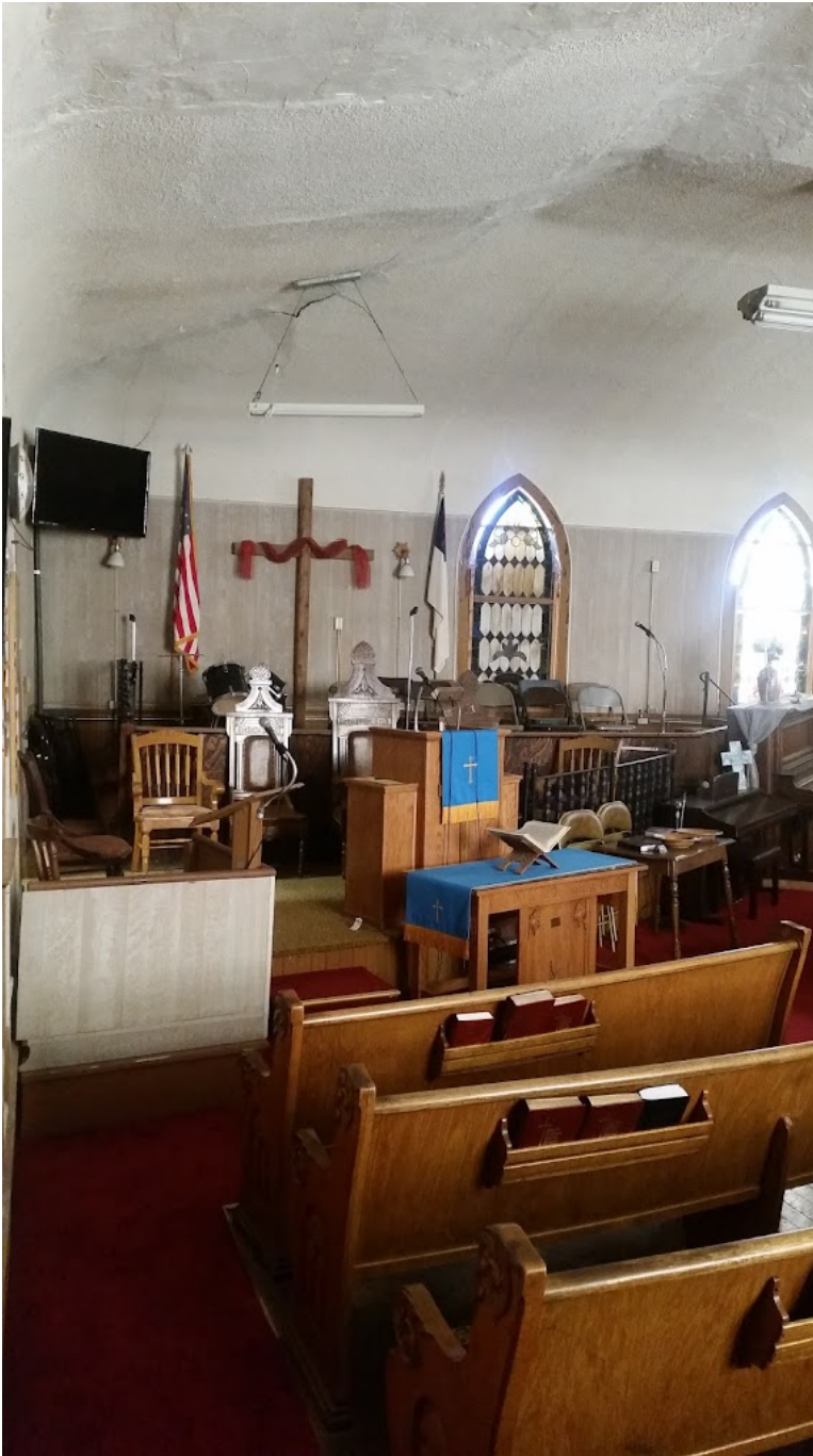
Figure 24: Sanctuary. View toward elevated pulpit and choir seating at southwest corner. 2019 photograph. Camera facing northwest. (Rev. Steve Mack)
