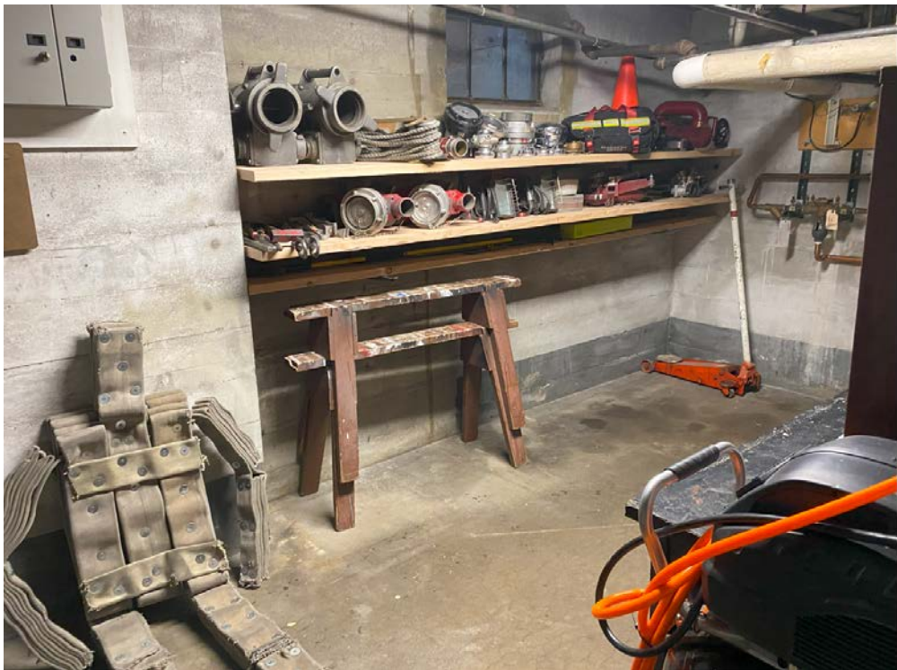
Photo 28: Storage room in basement, near southeast corner of the building.
