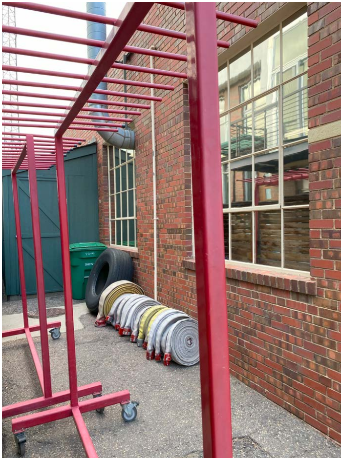
Photo 14: North façade of building taken from northwest corner.
