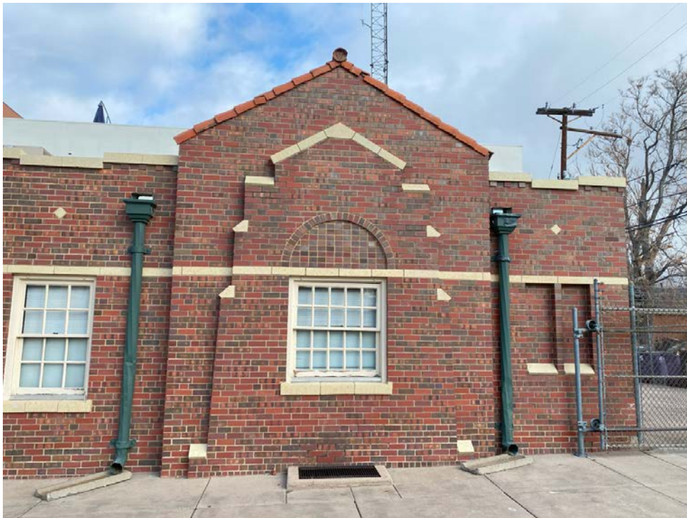
Photo 10: Close-up of south façade with gabled parapet on southeast corner of the building along 25 th Avenue.
