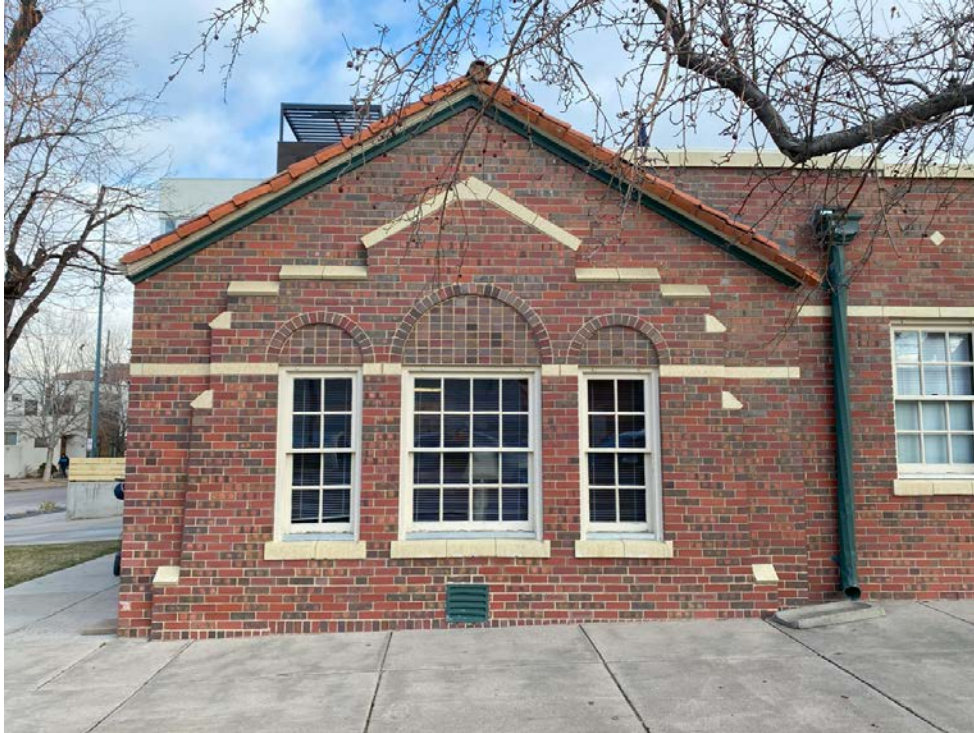
Photo 7: Close-up of south façade with gabled roofline on southwest corner of the building along 25 th Avenue and Washington Street.
