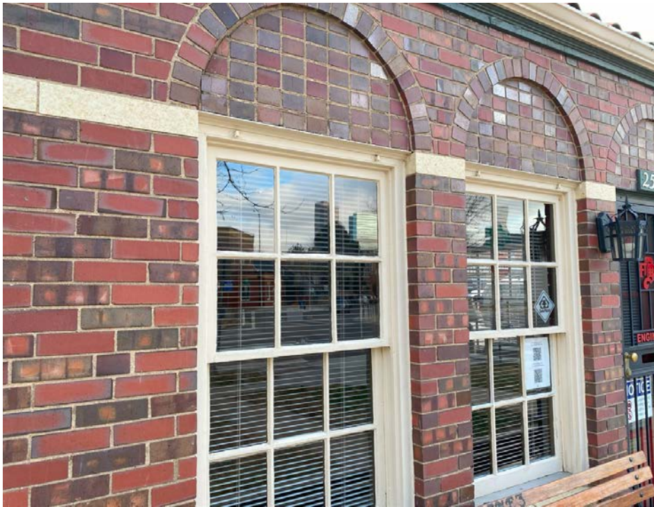
Photo 6: Close-up of front façade (along Washing Street) windows. Front door is visible to the right.
