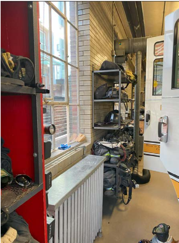
Photo 18: North interior wall of engine room. Three windows are located on the left side. The third window is blocked by a new structure (storage shed).
