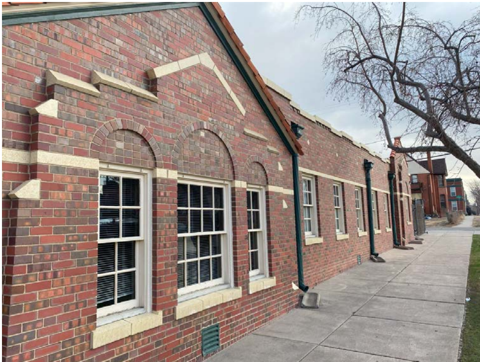
Photo 8: South façade (along 25 th Avenue) from southwest. The alley is visible in the distance.
