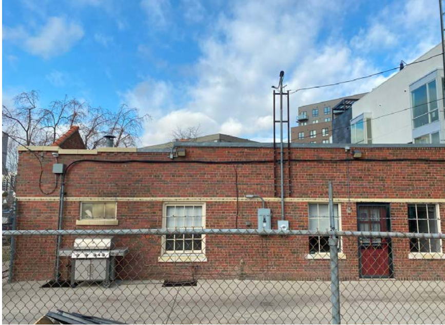
Photo 11: East façade of building with rear door visible. Photo is taken from the alley.
