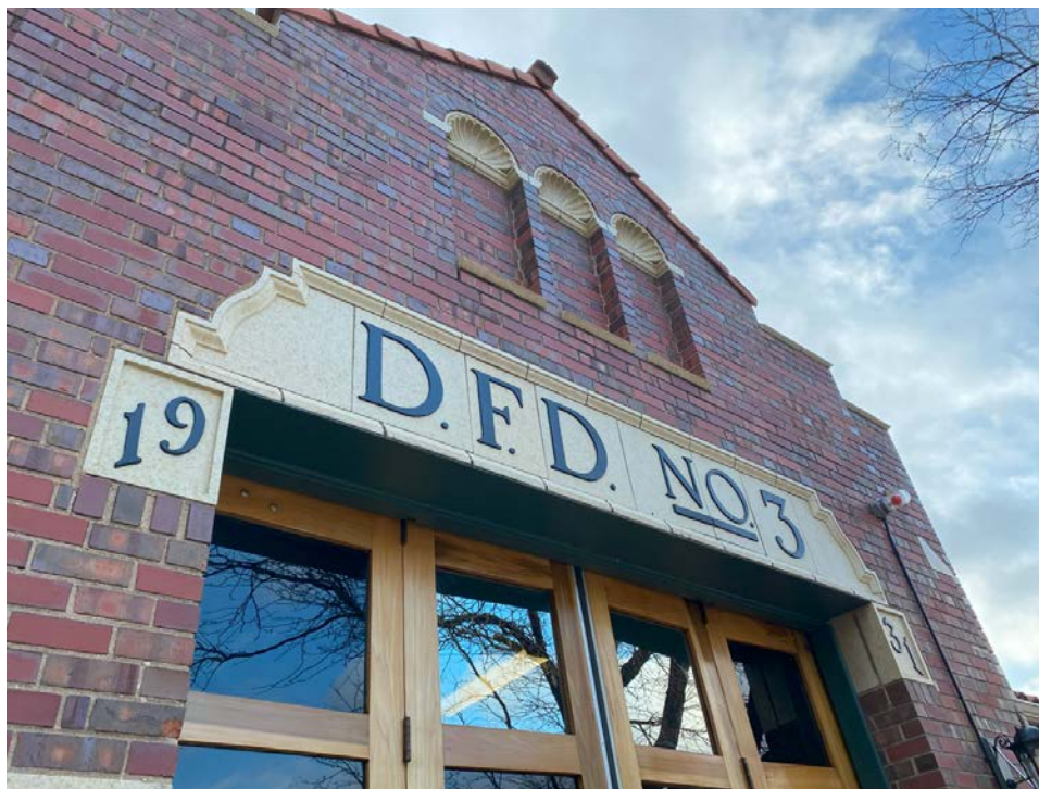
Photo 3: Close-up of gabled section of engine room exterior. Photo looking southeast.
