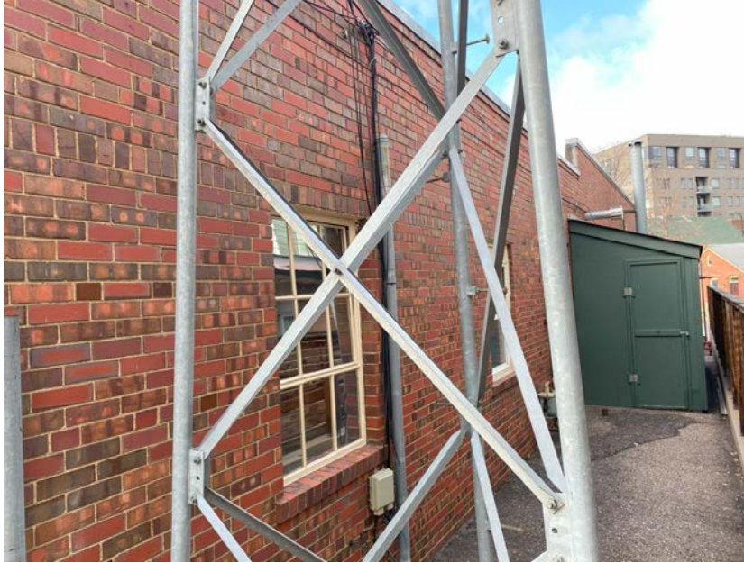
Photo 13: North façade from northeast corner of building (near alley). The base of the communication tower is in the foreground.
