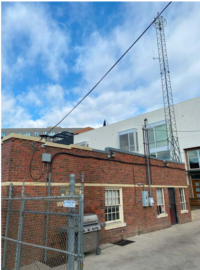
Photo 12: The east façade (rear of building) with communication tower visible. Photo taken from southeast corner of building.
