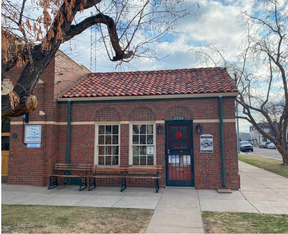
Photo 5: Close-up of front entrance and office windows located on the southeast corner of the building, along 25 th Avenue and Washington Street.
