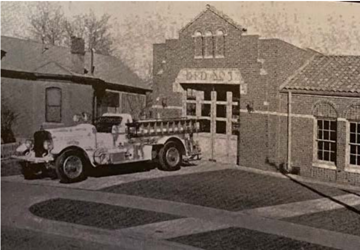
Figure 5: Engine in front of Fire Station No. 3 circa 1931. From the Denver Firefighter Museum.
