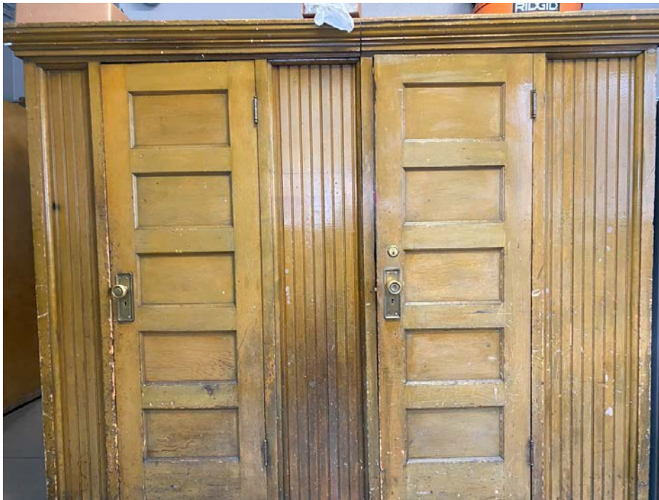
Photo 26: Wood closets in rear entry room.
