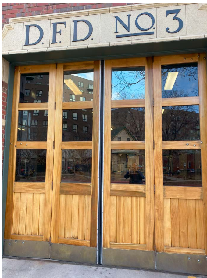
Photo 4: Exterior view of engine room doors (north façade along Washington Street).
