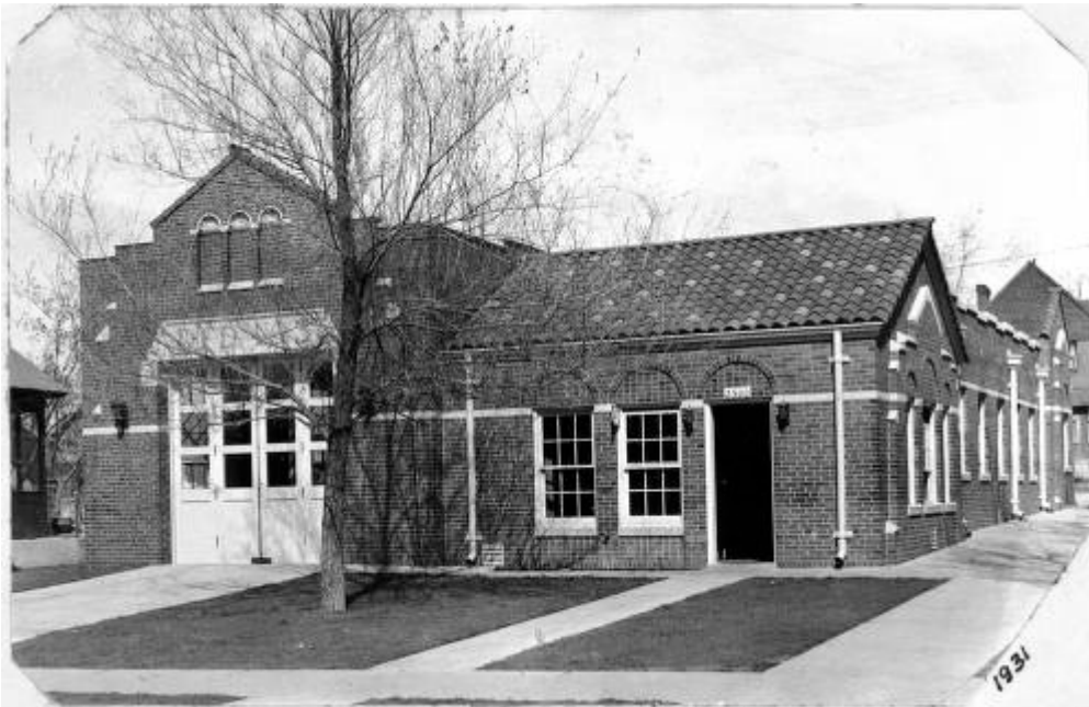
Figure 4: Fire Station No. 3 circa 1930s. From the Denver Public Library.
