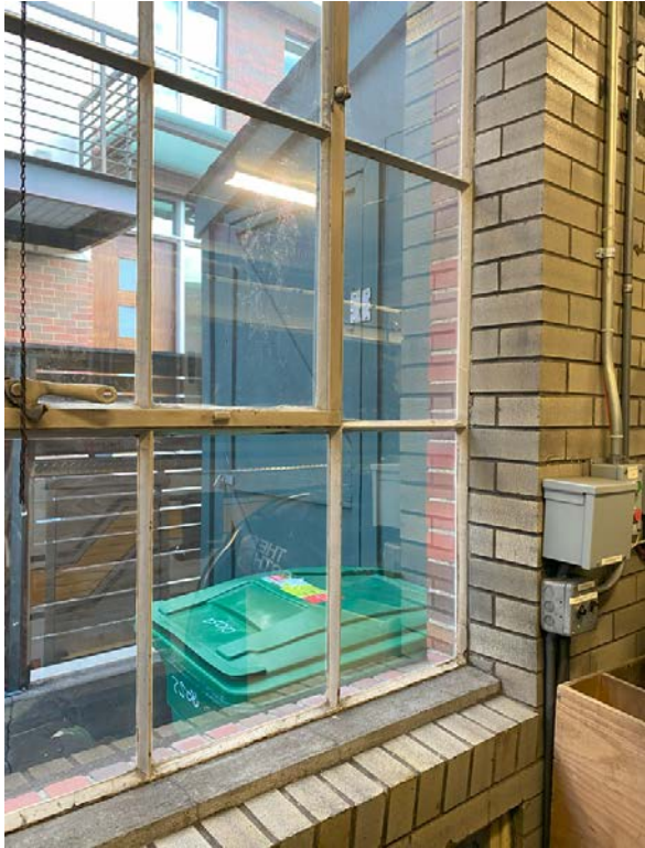
Photo 19: Close-up of middle engine room window on north wall. New storage structure is visible.
