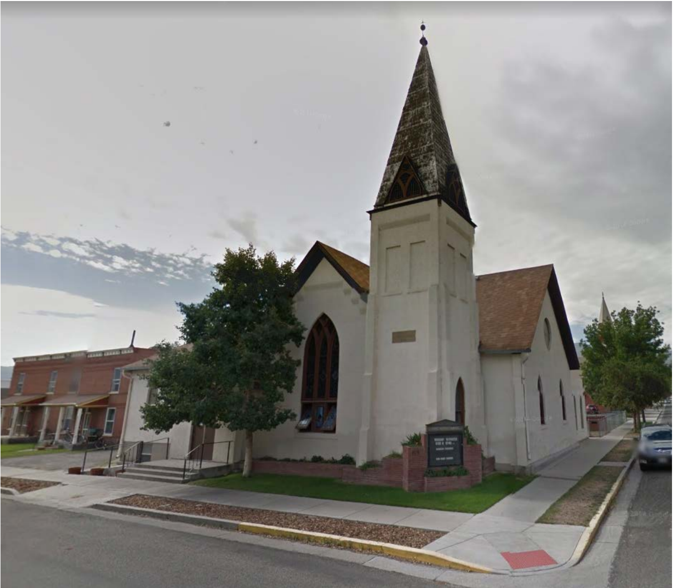
Figure 7: North and west sides in September 2012. Note stained-glass pivot windows added to the Gothic Revival stained-glass window on the north side in 1914. (Google Streetview)
