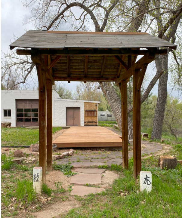
Photo 1: Entry gate, looking north.
