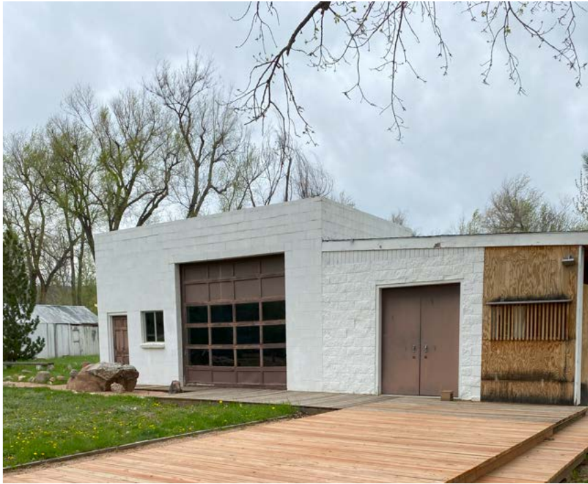
Photo 3: South façade on Indoor Practice Hall, looking north.
