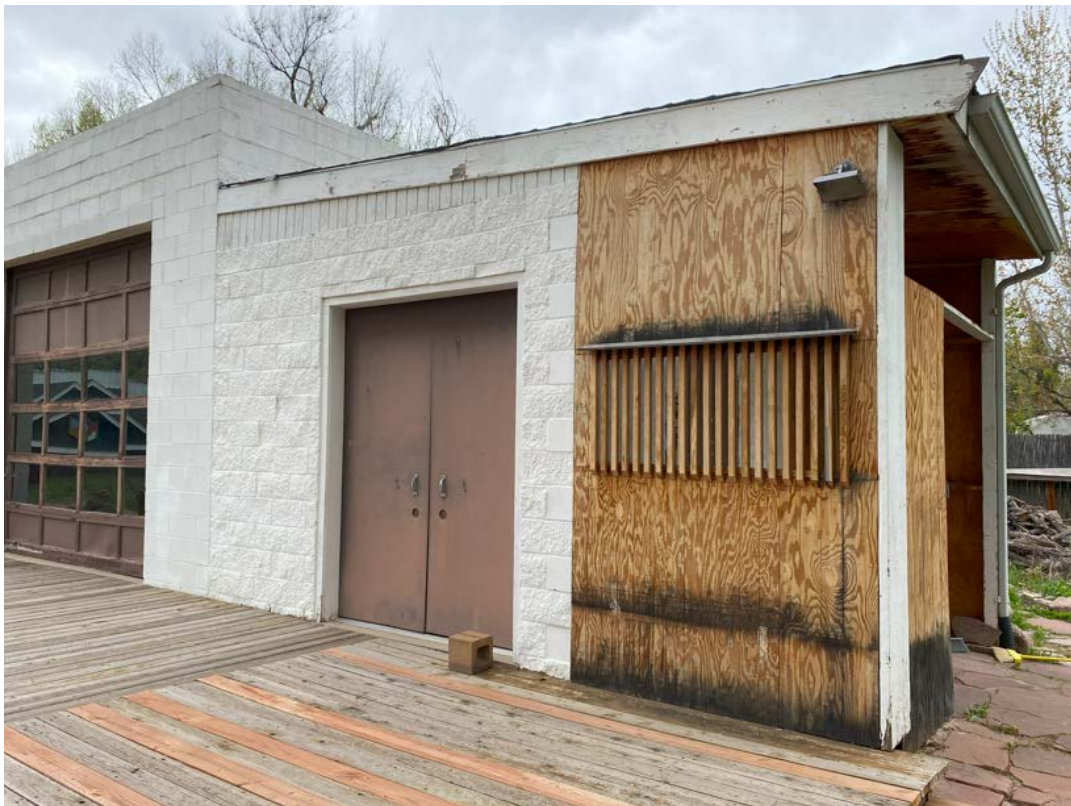
Photo 6: Looking north at Indoor Practice hall extension and entryway.
