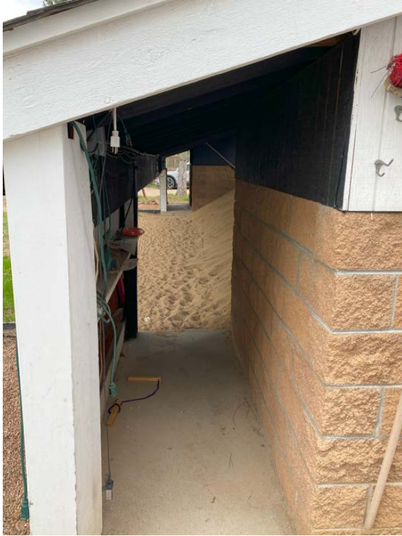
Photo 15: North entry, looking south, into target area.
