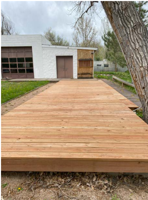
Photo 2: Platform, looking north.
