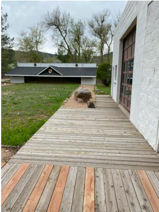
Photo 5: Looking west along western section of platform.
