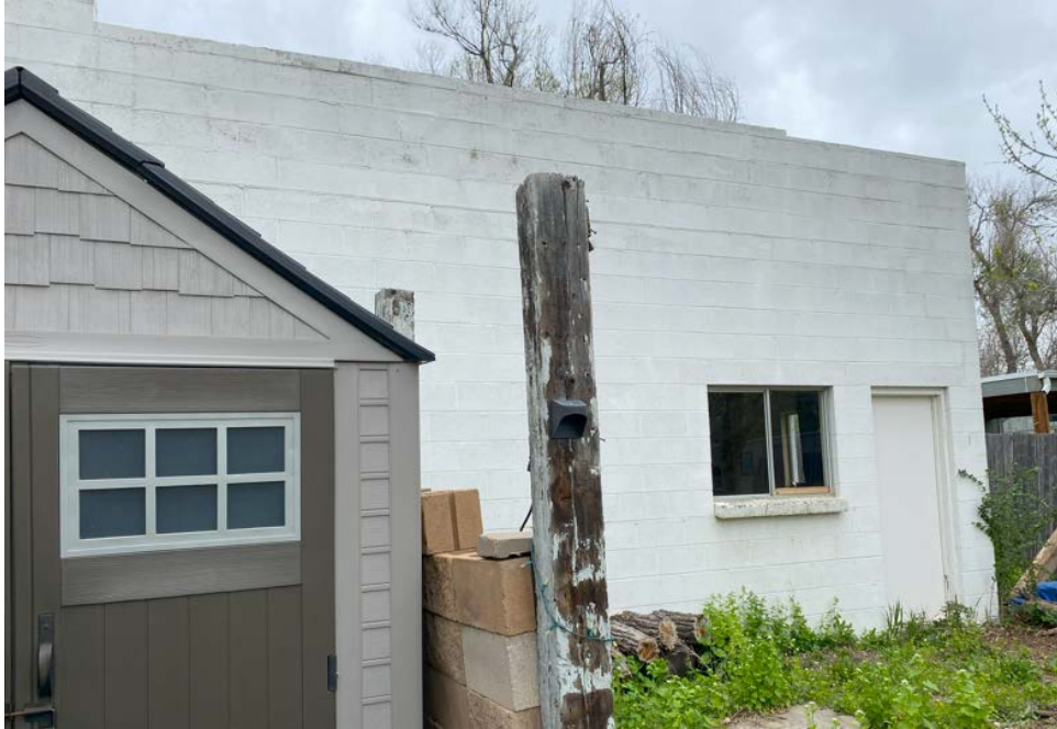
Photo 7: East façade of Indoor Practice Hall.
