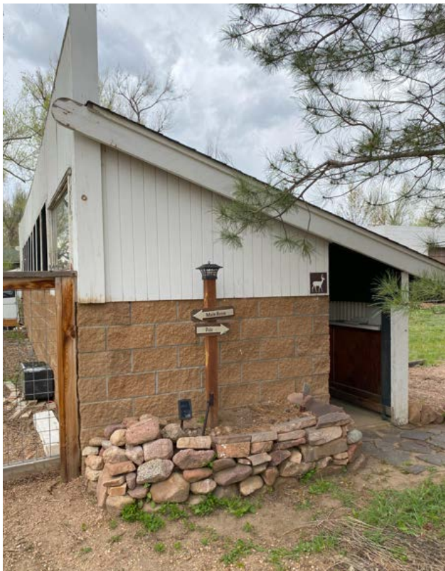
Photo 18: South entrance to the target area, looking north.
