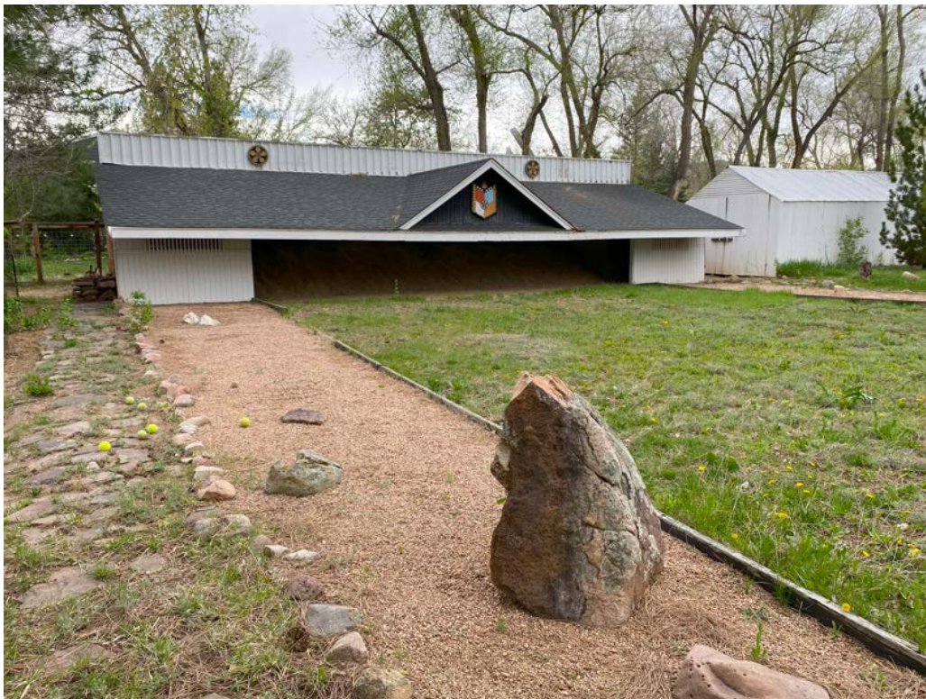
Photo 20: East façade of the target area.
