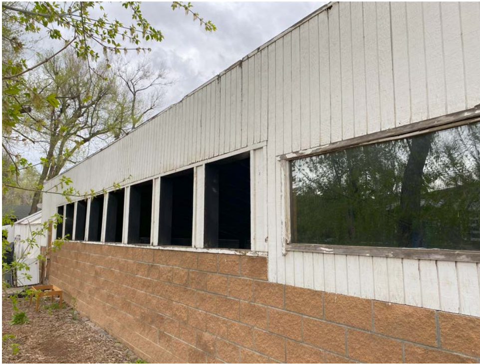
Photo 19: West façade of the target area.
