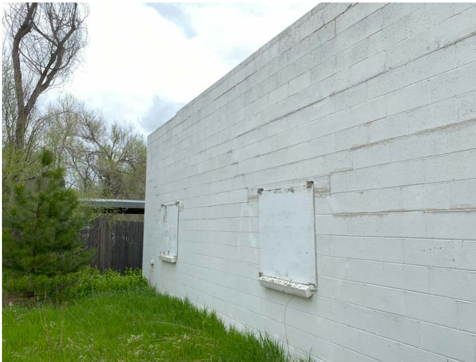
Photo 8: West façade of Indoor Practice Hall.
